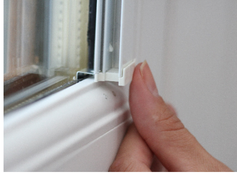
13. Engage the side extrusion bottom bracket into the bottom corner fixing bracket.
